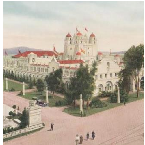
The California Building at the Panama-Pacific International Exposition; note that towers' design was inspired by the Santa Barbara Mission.
